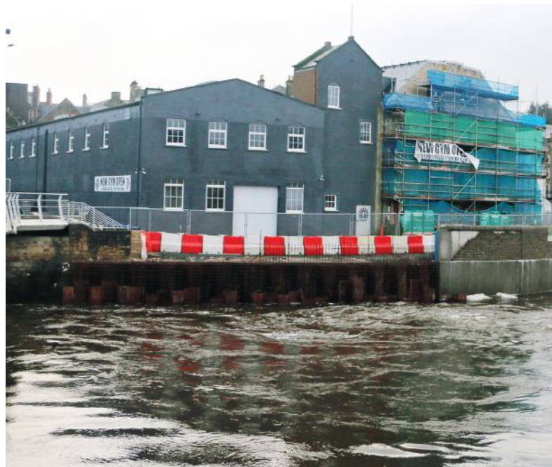
The temporary defences in the Mill Port area
